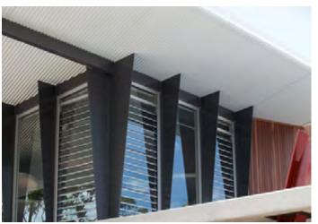
Key to the building's design were a series of vertical steel blades that required windows with a width of around 1400mm between them to achieve the desired aesthetic. Safetyline Jalousie was the only louvre window option available that could fulfil the width required. That width, along with the unique horizontal bars complemented the overall design.
